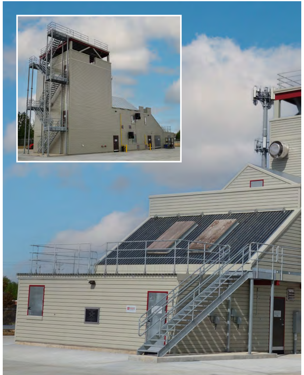
▲ Bentonville, Arkansas. This custom commissioner model tower is 30' wide and has 1
