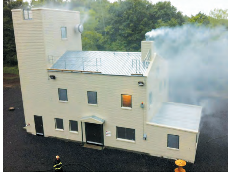
▲ The Town of Onondaga's Fire Training Center features an extra wide footprint with an exceptionally realistic residential interior layout.
