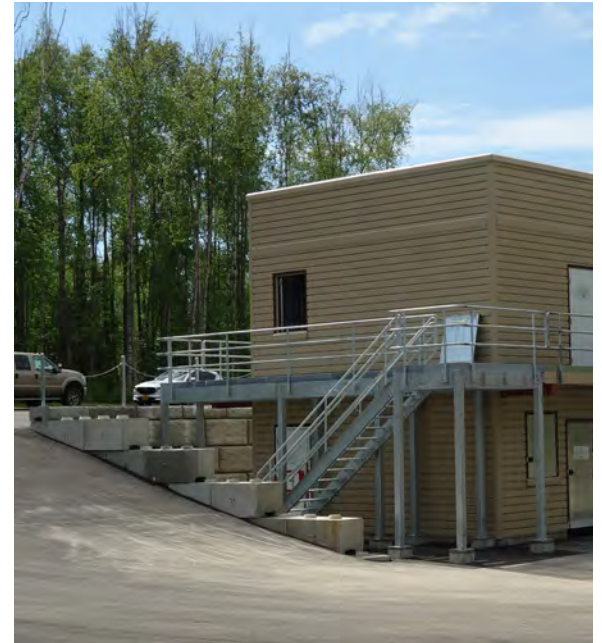
▲ Wasilla, Alaska- This Hall Crawler was built into basement entry.
