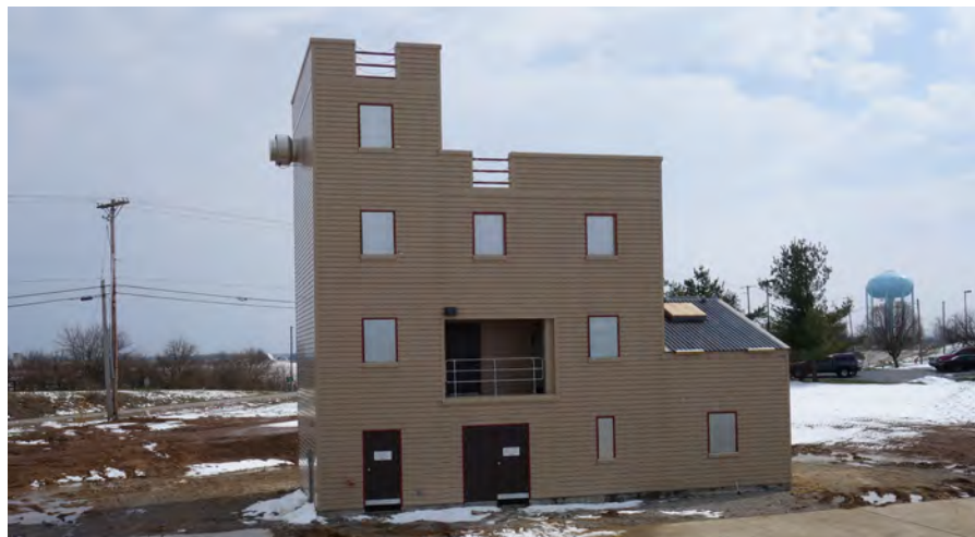
▲ Winchester, Kentucky- This Assistant Fire Chief model has a 3-story residential section and has an off-set gabled roof over the annex portion of the tower.
